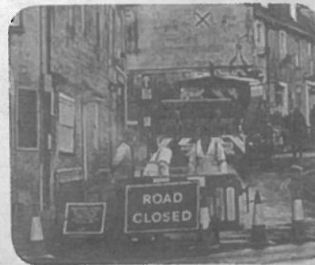
5 Repairs to streets and freeways. (4, 4)
